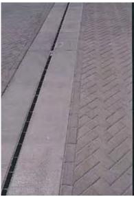
Cutting pavers to fit at the drains used units no smaller than one third of a paver.
