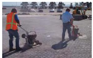
Initial compaction of the pavers in the bedding sand was done on large areas at one time.
