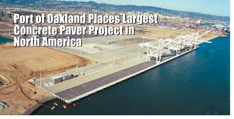
Berths 55/56 at the Port of Oakland utilizes a record breaking 39 acres (16 ha) of interlocking concrete pavement for container yards. The earth works in the right background (behind cranes) will see an additional 46 acres (19 ha) next year, soon to be another record breaker.
