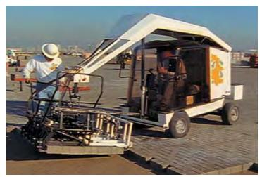
Mechanized equipment lifts and places several paver layers per minute.
