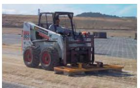
Joint sand is swept across the paver surface and into the joints. A second compaction (not shown) with plate compactors help move the sand into the joints. The paver surface was later proof rolled with a large roller to further seat the units into the bedding sand.
