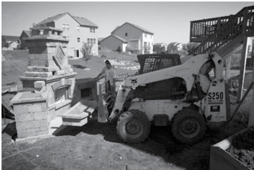
Figure 6-13: Hearth module is placed in front of fireplace.
