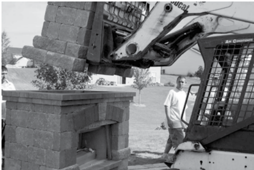
Figure 6-11: Chimney module is stacked on top.
