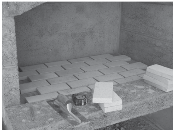
Figure 6-7: Fire brick is installed on the interior of the fire box.
