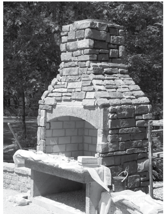
Figure 6-8: The exterior of the fireplace is covered in this case with cast stone veneer.
