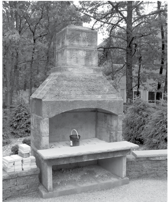
Figure 6-6: Precast elements are assembled on site.
