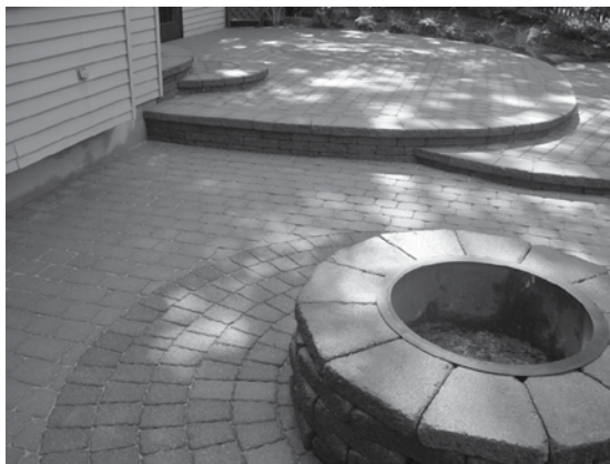
Figure 6-4: An example of a fire pit lined with a steel sleeve.
