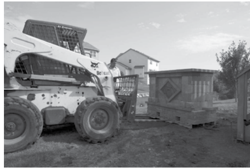
Figure 6-10: First module is placed on base.
