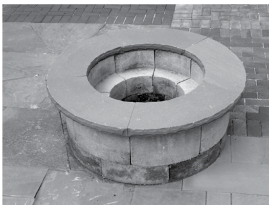
Figure 6-5: This fire pit is cast from heat resistant concrete and can be covered with different materials to match the project.
