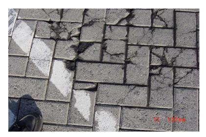
Figure 1. Showing typical damage under corner castings. This type of damage has caused no loss of service.
