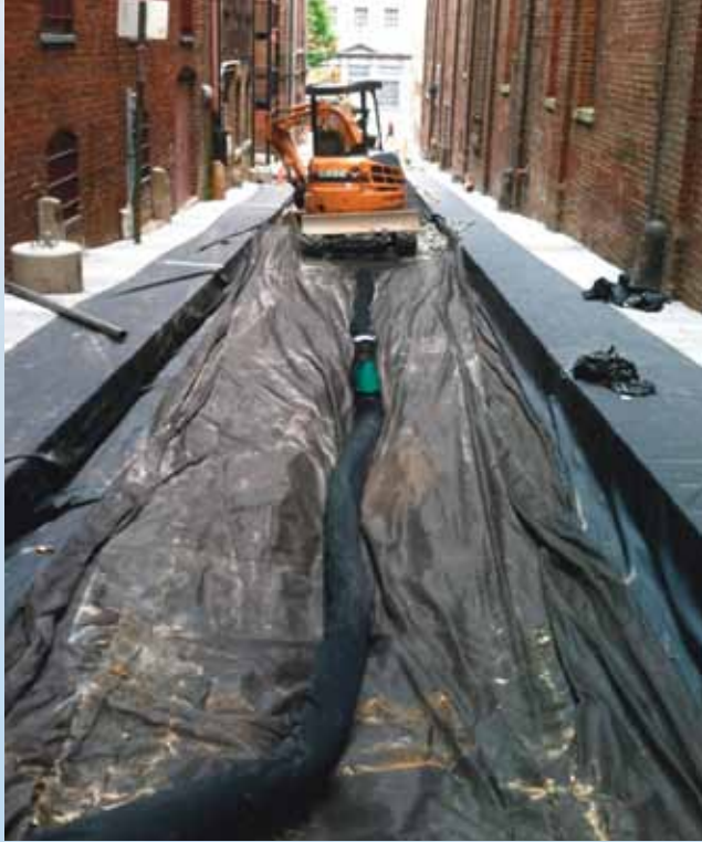
Figure 2. Geotextile is placed over a geomembrane for protection against the aggregate subbase in a green alley in downtown Richmond, VA.
