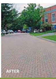
With its construction completion first reported in November 2010, the PICP drive and parking lot monitored by the University of New Hampshire Stormwater Center captured almost all rainfall without outflows from the base.
