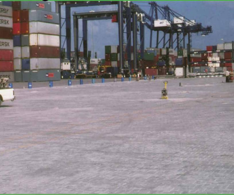
Civil Engineers that specialize in heavy-duty pavements choose LIQUID STABILIZER'S on their projects. Liquid stabilizers offer long lasting "cured" stabilization with greater consistency in the sand joints on the entire project. Liquid stabilizers also stabilize joint sand with the correct gradation and quality and can be installed at a rate of more than 10,000 square feet per hour. Most importantly, this quality does not cost you more money on your next project.
