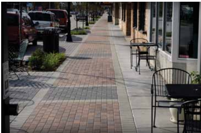
Sidewalks combine PICP along to allow water to soak into the structural soil under the trees while regular ICP is built with a 8 in. (200 mm) thick compacted aggregate base.
