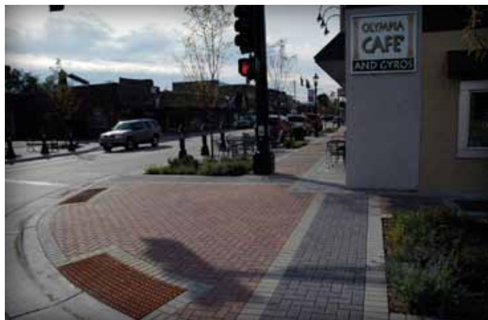
Cast iron detectable warnings set in concrete accent curb ramps.
