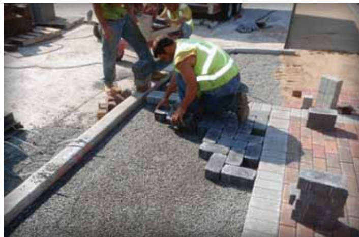
Granite chips are used under the PICP and bedding sand under the ICP in the sidewalks.
