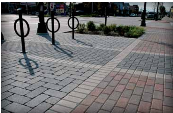
Sidewalk pavement under these bike racks combines permeable units with regular pavers to feed the street trees.
