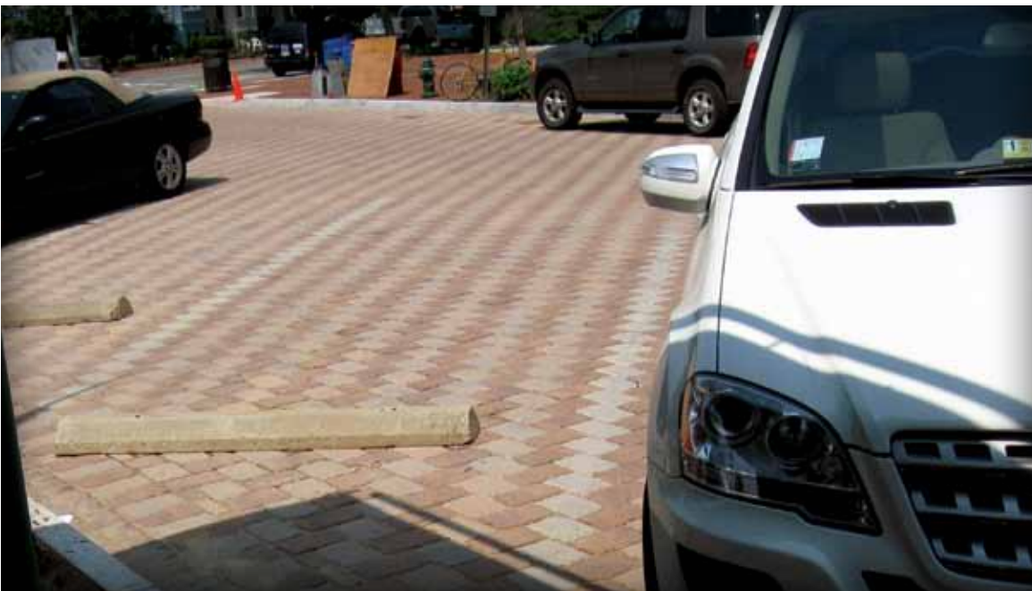
Gray pavers in the herringbone paving pattern mark parking stalls in front of the Eastern Market building. No paint or repainting required.
