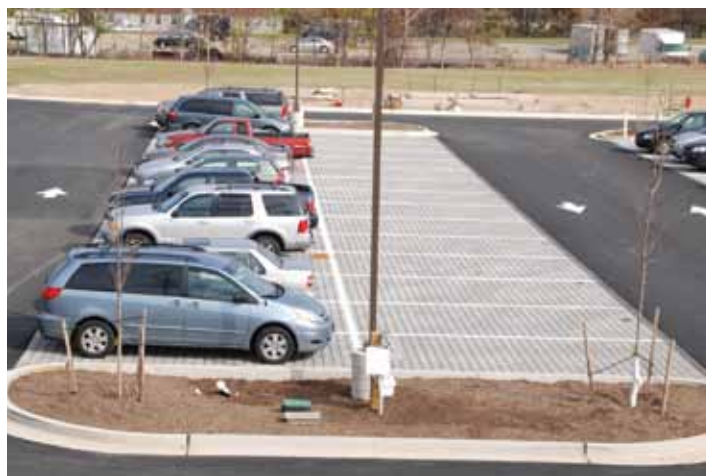
The new parking lot replaced an old concrete floor remaining from a demolished World War I building. The 5,230 sf (494 m 2 ) PICP test section at right was supplied and installed by ICPI members.
