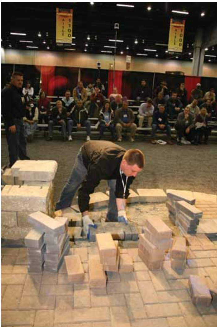
Raised paver and SRW patio construction is demonstrated at the Hardscape North America show
