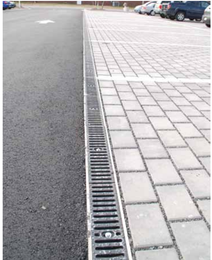
PICP and impervious asphalt are separated by a slot drain to collect runoff from the asphalt and compare it to the PICP infiltrate.
