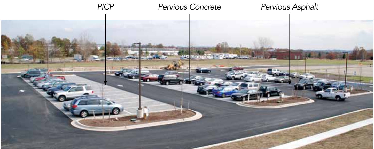
The EPA employee parking lot includes similar sized PICP, pervious concrete and porous asphalt test areas separated by impervious asphalt driving lanes. Runoff from the asphalt will be compared to that from the permeable surfaces.
