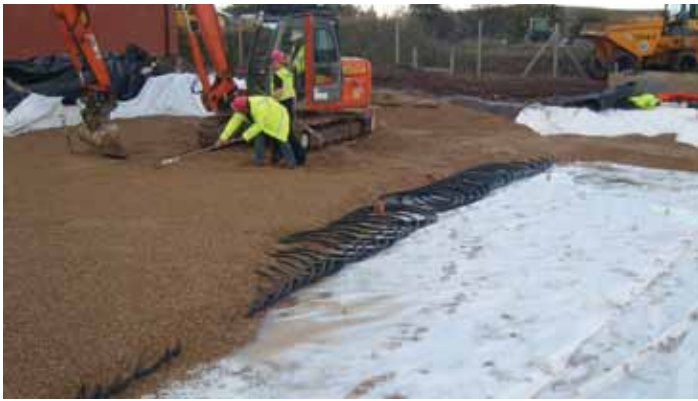
Construction of a PICP parking lot in the UK using ground source heat pump technology to support building heating and cooling. The coiled pipes provide a heat exchange with water stored long-term in the PICP base. Photo provided with permission from Hanson Formpave.
