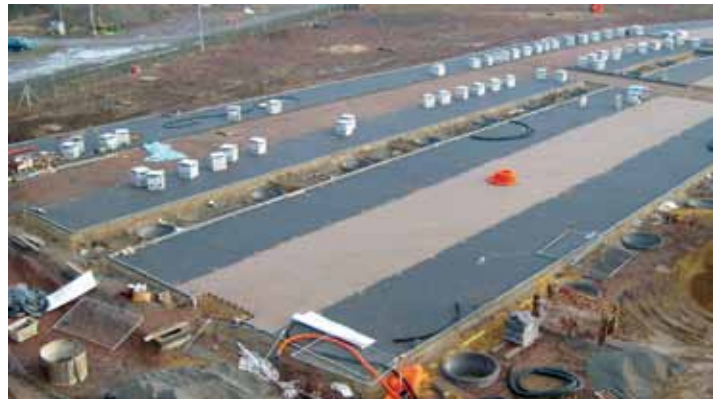
The same PICP parking lot in the process of receiving concrete paving units. Photo provided with permission from Hanson Formpave.
