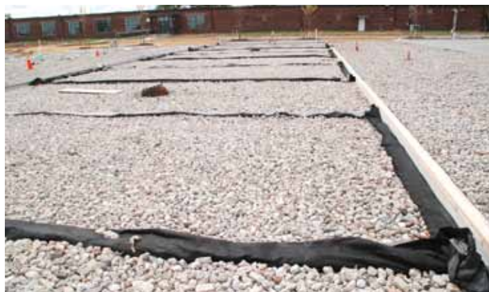
Crushed, washed and graded No. 2 subbase was recycled old concrete. The black flaps protruding from this material are the impermeable liners used in alternating areas. The liners are also lined with geotextile for projection.
