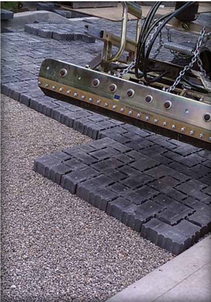
Figure 3. Now the norm for PICP installation, machine assisted paver placement accelerates installation time compared to manual methods. The pavers were installed by an ICPI member.
