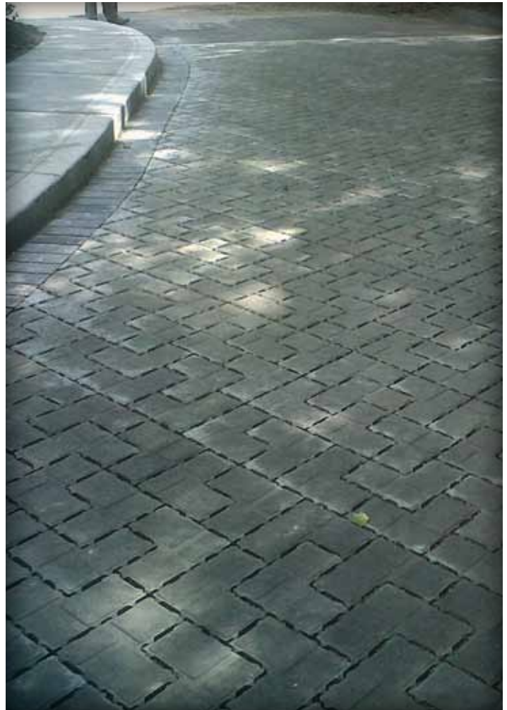
Figure 4. The finished surface shown here comes as a result of filling the paver joints with No. 8 stone, sweeping, then compacting the paver surface.
