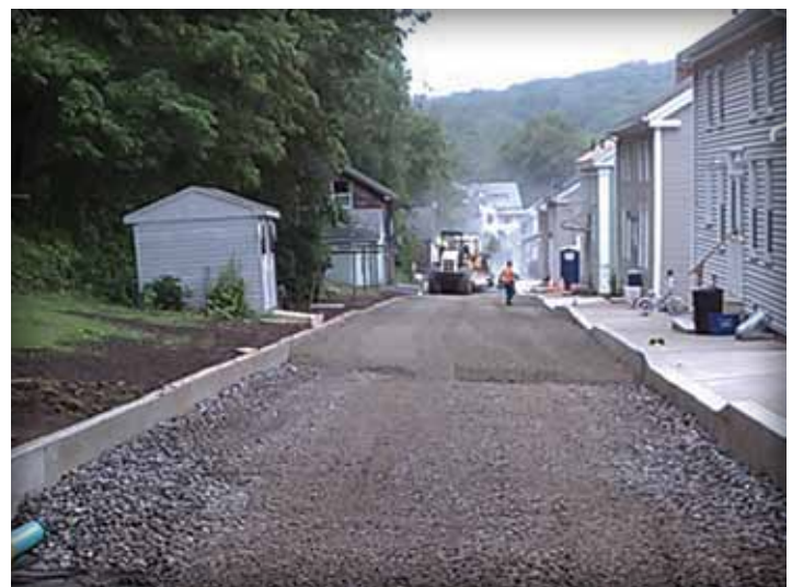
Figure 2. This view illustrates the installed ASTM No. 2 stone under the No. 57 layer with a drain pipe along one side of the road.
