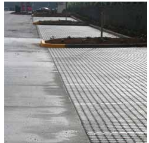
Figure 11. PICP and poured-in-place concrete meet. A best practice is to separate the bases between these two pavement systems with an impermeable liner.
