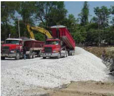
Figure 2. Elmhurst College in Elmhurst, Illinois used very thick bases to accomplish underground detention/infiltration for landscape irrigation in certain parts of a large PICP parking lot. The thick bases provided additional structural support for heavy trucks.
