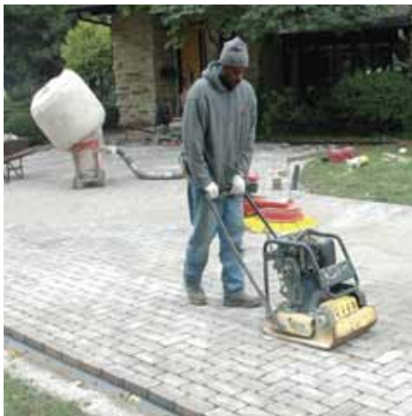
Figure 9. A plastic edge restraint is nailed into the compacted, dense-graded base material. Permeable pavers are installed per manufacturer and ICPI recommendations.
