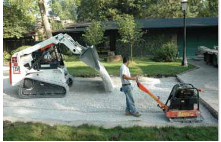
Figure 8. Both bases—dense-graded and open-graded—are compacted to the same elevation.
