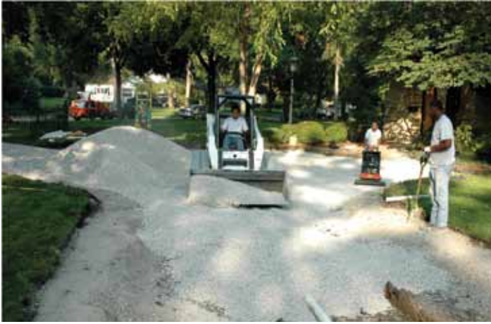
Figure 7. Dense-graded aggregate base material forms berms along the sides of this PICP residential driveway. Open graded aggregate base is placed in the center to store and infiltrate water.
