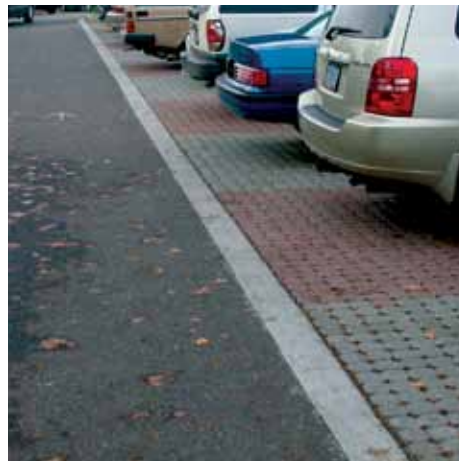
Figure 10. PICP that meets asphalt should be separated with a concrete curb or beam.
