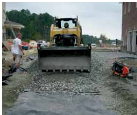
Figure 3. Equipment spreading aggregate and rides on the aggregate to keep it clean.
