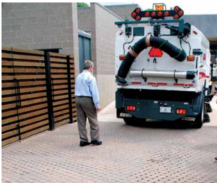
Figure 5. Vacuum equipment draws out dirt and soils stone from a PICP. The openings are refilled with stones. Such equipment would likely be required in removing dirt and sediment pressed into PICP openings during construction.
