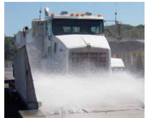
Figure 4. Truck washing equipment might be a cost-effective solution to keeping mud and sediment from PICP surfaces during construction.
