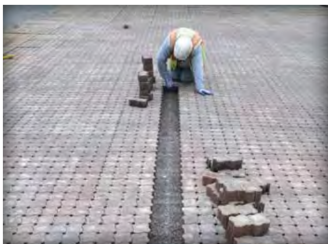
Figure 5. Prior to filling the joints with stone, pavers are removed and replaced with different color units to mark the parking stalls. This eliminates painting stripes.
