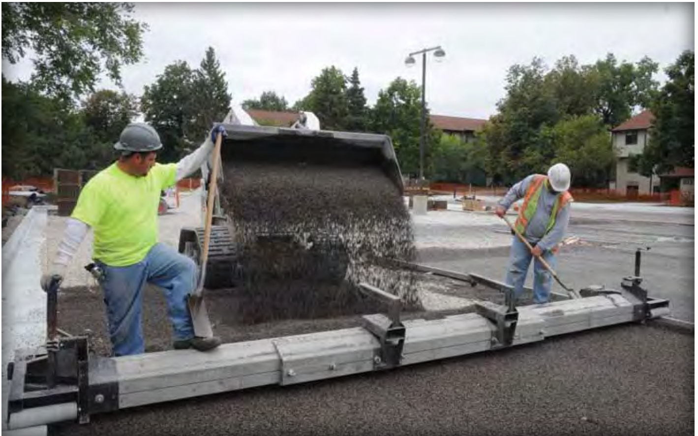
Figure 2. A wide screeding machine or screed "bucket" enables smoothing of the No. 8 stone bedding material prior to placing the concrete pavers. Note that one side rides on the existing concrete curb and the other on a metal screed rail.
