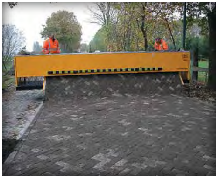
Tiger Stone rolls out a concrete carpet with their paver installation equipment.
