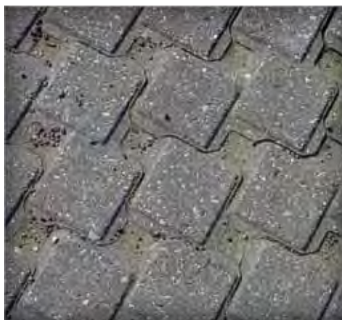
Figures 4 and 5. Before and after cleaning with fresh stones swept into the joints
