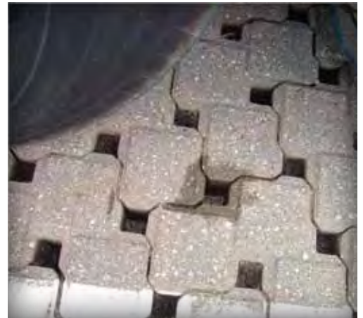
Figures 2 and 3. The vacuum machine removed the top inch (25 mm) of sediment and jointing stone.
