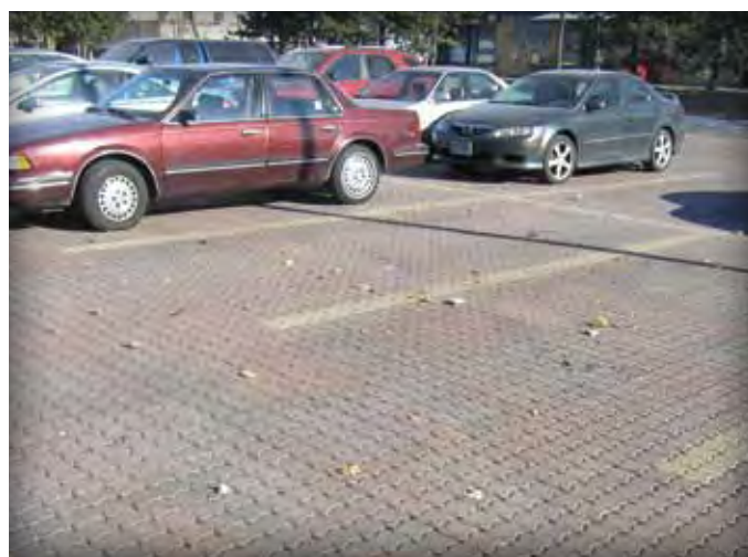
Figure 6. The finished PICP surface with parking stalls marked with colored pavers
