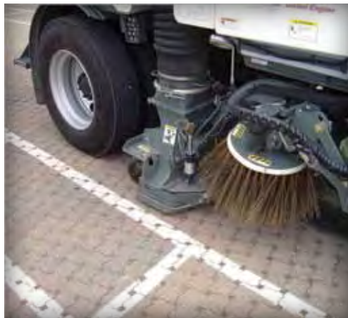
Figures 2 and 3. The vacuum machine removed the top inch (25 mm) of sediment and jointing stone.
