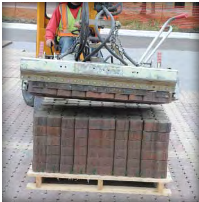
Figure 3. Lifting a layer of concrete pavers from the shipping pallet with an installation machine and clamp
