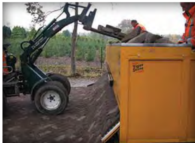
Figure 4. A loader rides on the newly paver concrete pavers to load more pavers into the machine's hopper.
