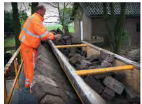
Figure 3. Those aren't tumbled pavers. Sustainable paving is normal in The Netherlands meaning that concrete pavers get reused at every opportunity for low-speed vehicular pavements.
