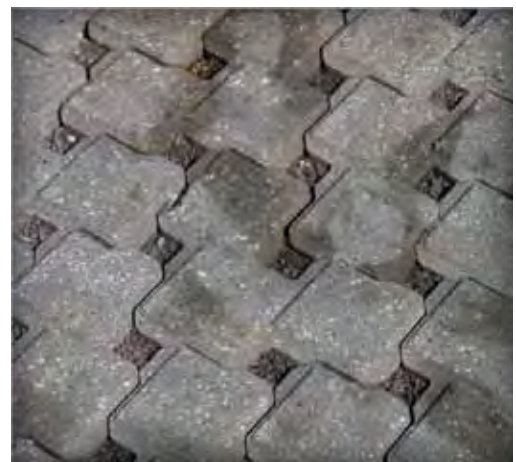
Figures 4 and 5. Before and after cleaning with fresh stones swept into the joints
