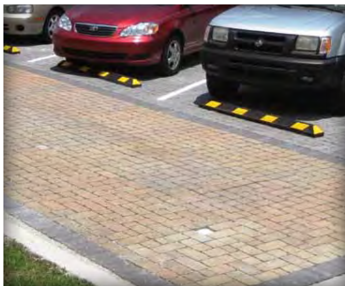
Figure 7. A PVC pipe with a screw cap serves as an observation well on PICP parking lot at a U.S. Army base in Georgia.
