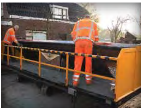
Figure 1. Rather than leaning over, workers stand on the machine while it moves on the bedding sand on treads.
